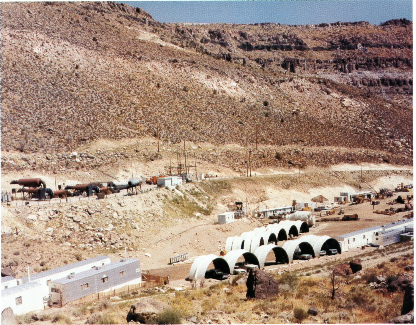
FIGURE 12-33. DIAMOND SCULLS PORTAL AREA SHOWING LARGE PIPE SECTIONS TO BE ASSEMBLED IN THE TUNNEL FOR SPARTAN MISSILE SURVIVABILITY TESTS
